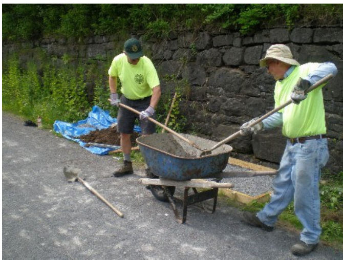
Dave Wright and Chauncy Young mixing cement for a pad.
